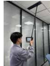
ceiling duct inspection
